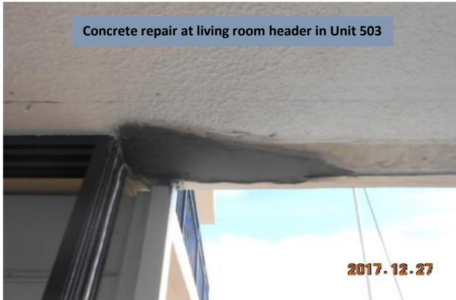
Concrete repair at living room header in Unit 503
