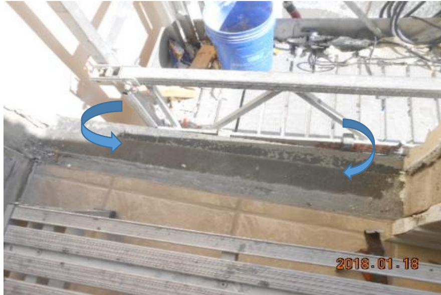
Photo shows recently cast sill at east guest bedroom window, Unit 2003
