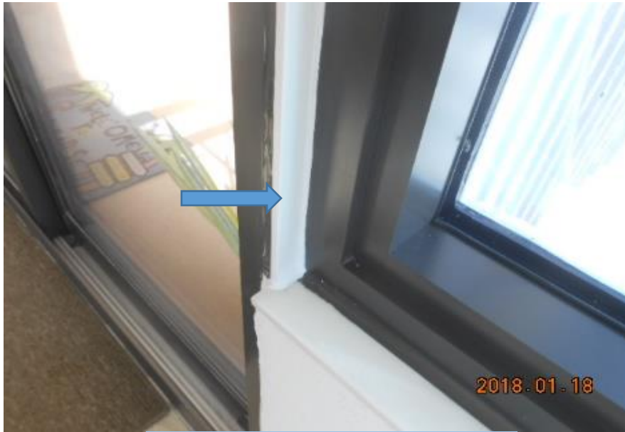
Lattice trim piece at window juncture
