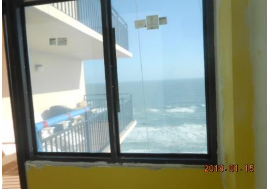
Window install at east living room window in Unit 2103
