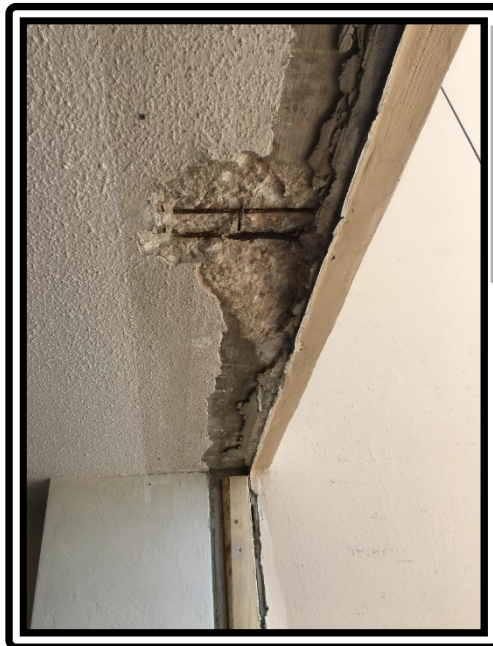
View of Unit 603 guest bedroom header excavation
