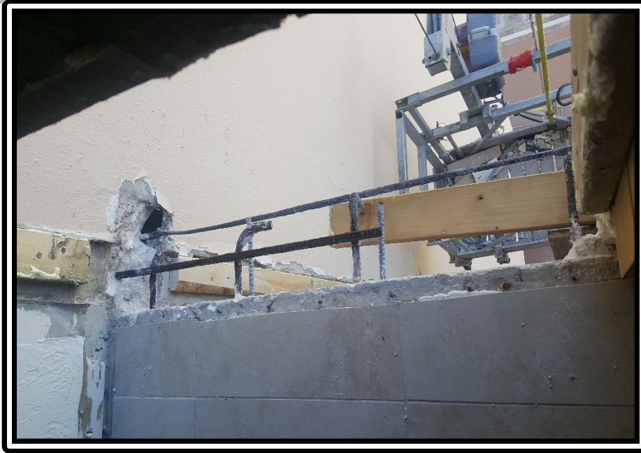
Unit 603 header / Unit 703 guest bedroom sill excavation
