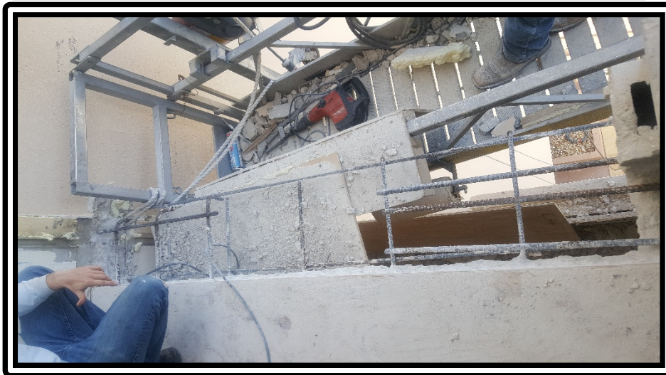
Unit 703 guest bedroom excavation of knee wall
