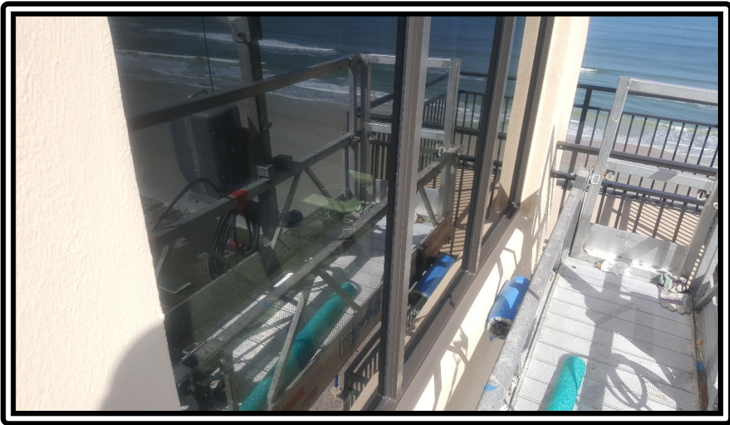
02 Stack living room south 3 section fixed window walls painted
