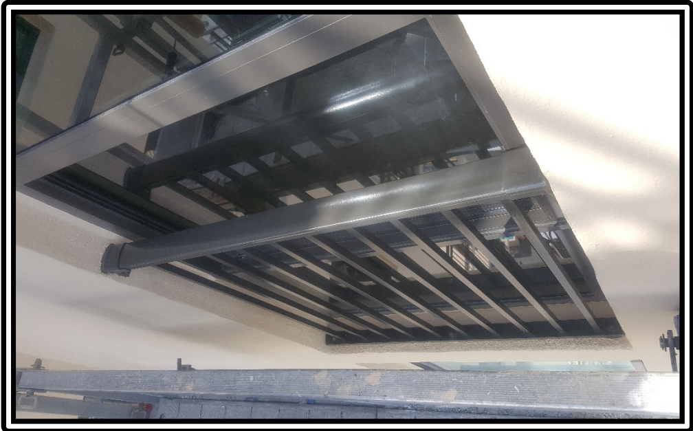
02 Stack window walls painted
