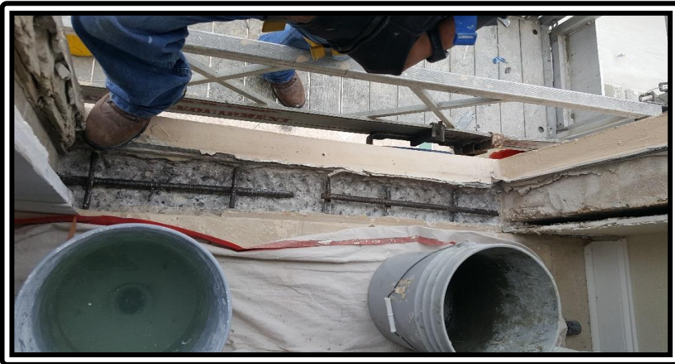
Concrete excavation and repairs in master bedroom Unit 2003
