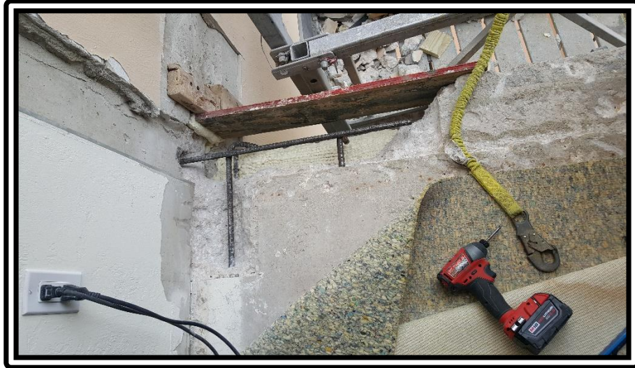
Unit 503 guest bedroom concrete excavations and repairs on floor
