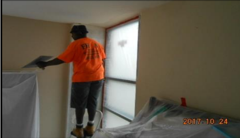
Plaster work in progress in Unit 1801 master bedroom
